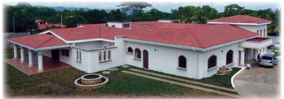
Construction of Centro Santa Inés, the Home that Love Built in Nicaragua for the elderly Sisters of St. Agnes, was initiated in January and completed in October 2010. Prudent stewardship and the generosity of friends and donors of CSA helped to offset a portion of the cost for construction of the facility.
